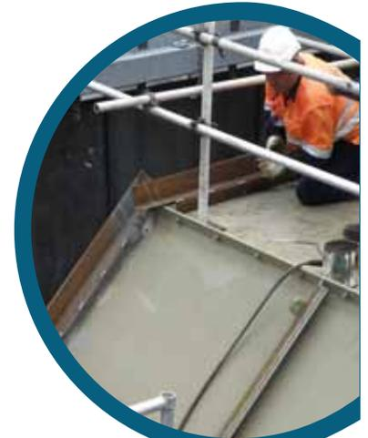
Preparing the breaker unit for installation of Hushclad
