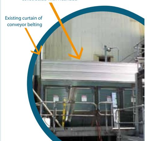
Acoustic enclosure lowering onto the drive end of Bradford Breaker
